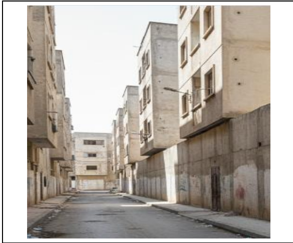
Figure 3: Blind frontages and high boundary walls eliminating "Eyes on the Street" and visual permeability.
