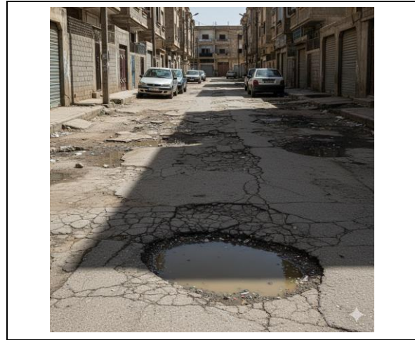
Figure 4: Level-zero morphology and surface degradation compromising tactile navigation and safe pedestrian boundaries
