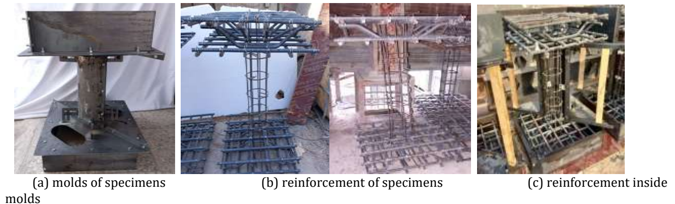
FIGURE 5. Molds of specimens and reinforcement details.
