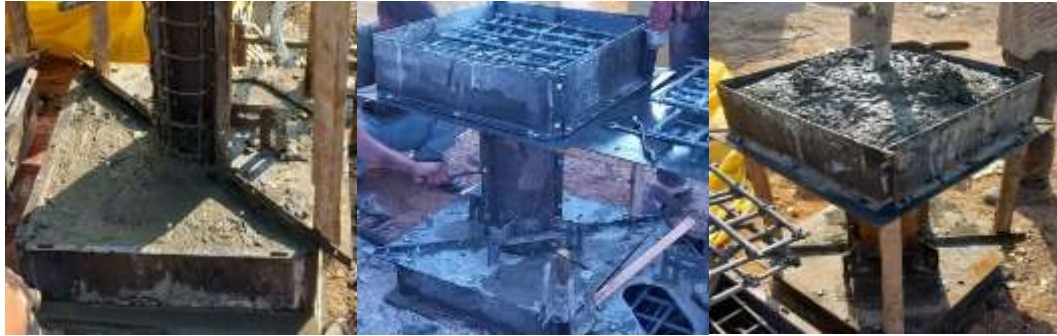
FIGURE 6. Stages of casting concrete for the specimens.
